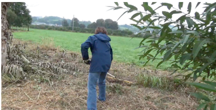
FIGURE 39: Maria clearing the surface grass.
